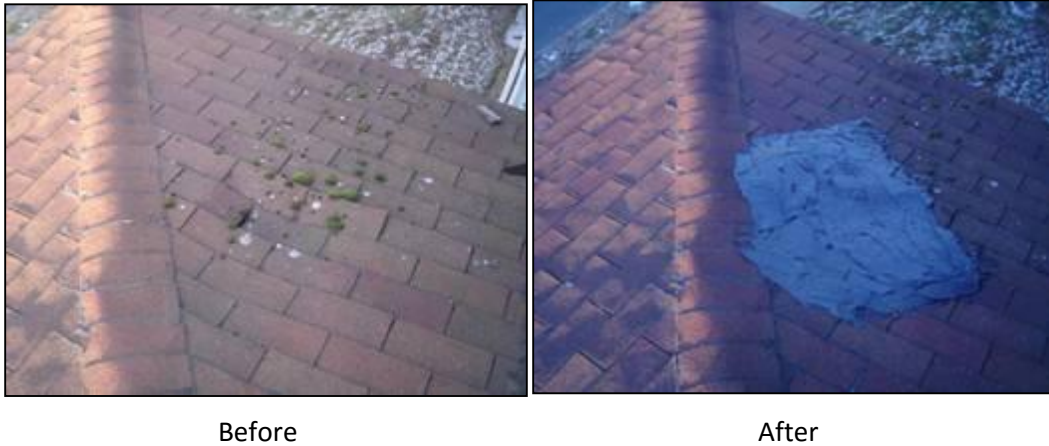
Figure XXIX: Sealing a roof
