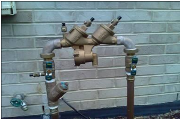
Figure X: Radiant system RPZ valve
