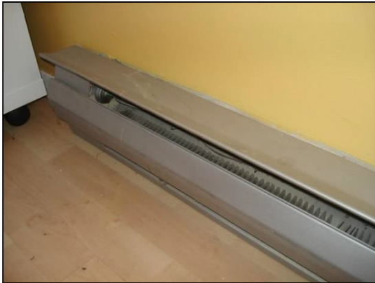
Figure IX: Radiant system baseboard
