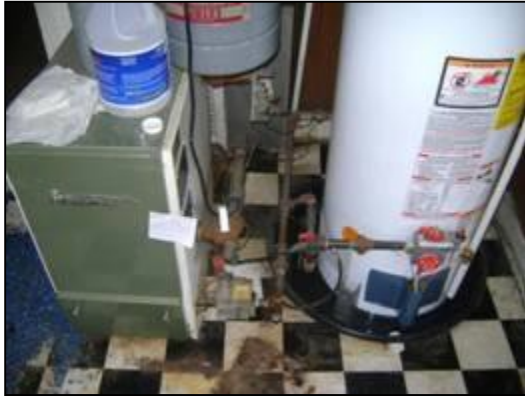
Figure VI: Steam system boiler
