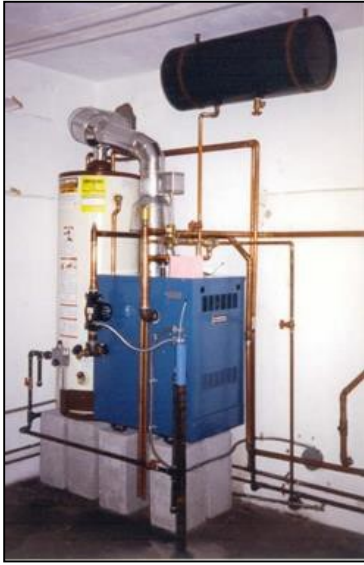
Figure VIII: Radiant system expansion tank
